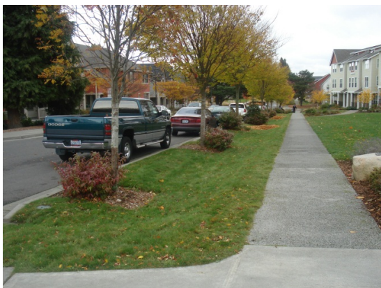
Figure 1 – High point, where major redevelopment of a residential area took place and the stormwater drainage is now predominantly managed on the surface. Here a shallow swale in the verge drains the highway.
