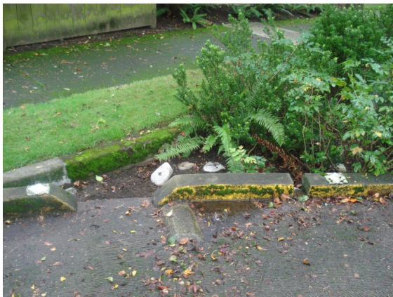
Figure 15 – Entrance detail to a street planter. Note the added raised shallow kerb to try and divert flow into it.
