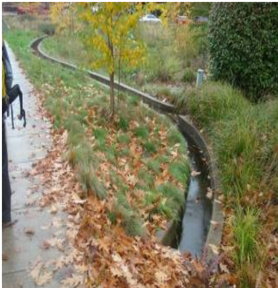
Figure 21 – Rill to take flow to a detention area fitting in with the local urban design.
