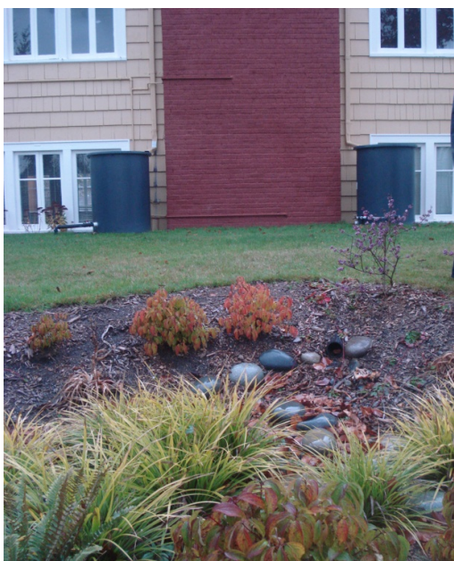
Figure 11 – Two cisterns intercepting downpipes on a large residential building. One discharges via a pipe to the raingarden and one via a covered stone trench.
