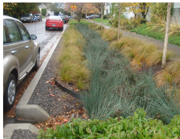
Figure 14 - bioretention area where a plastic strip (in the foreground to the left) was held in place by shallow wooden pegs, likely to degrade and break allowing stone against the kerb to fall away.
