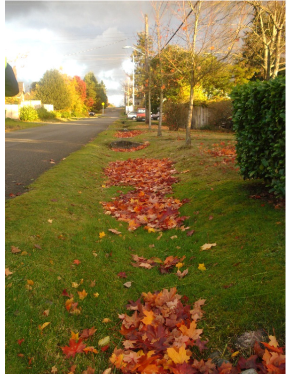
Figure 22 - Shallow swale in a street, with simple driveway crossing in the verge and trees in close proximity
