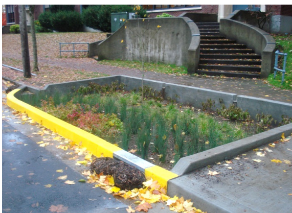
Figure 18 – street planter in Portland with yellow kerb to indicate no parking. Note the relatively high drop close to the exit from the school steps. Also the planting is protected until more substantially grown by the barriers in front of the inlets.
