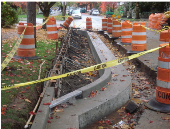
Figure 25— street planter in construction during the visit. This shows the updated design for flows to enter along the kerb line, and wider inlet to reduce blockage likelihood.
