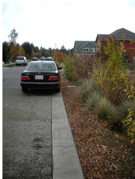
Figure 23 – Sloping carriageway towards a bio-infiltration swale
