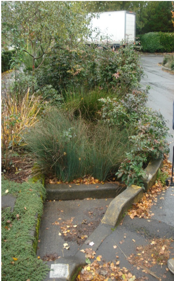
Figure 4 – Stormwater planter where the day to day maintenance is undertaken by the residents. They partially dictate the scale of plant growth.
