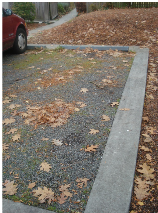
Figure 10 – example of porous paving for car parking in a redevelopment area
