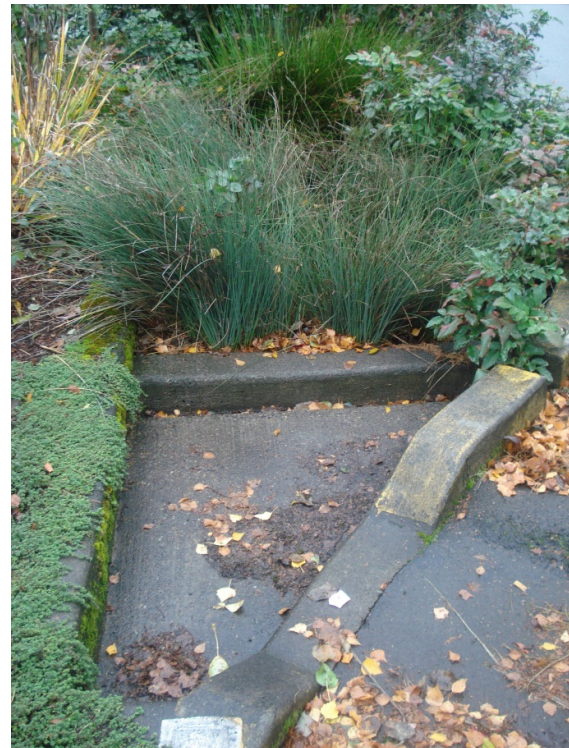
Figure 24— well established street planter inlet, with a concrete sediment bay. Note the re-profiling of the highway to divert flows into the planter.
