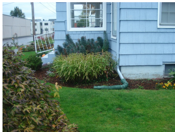
Figure 2 – Example of downpipe disconnection in Portland on a residential property.
