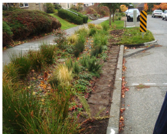
Figure 13 – Location where the measures had been removed. Note the kerb inlet blocked and recently filled in earth next to the kerb. Also, the hazard signs required in Seattle (top right).
