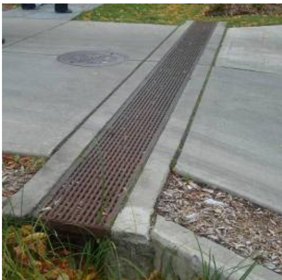
Figure 19 – Grated channel to pass flows under driveway
